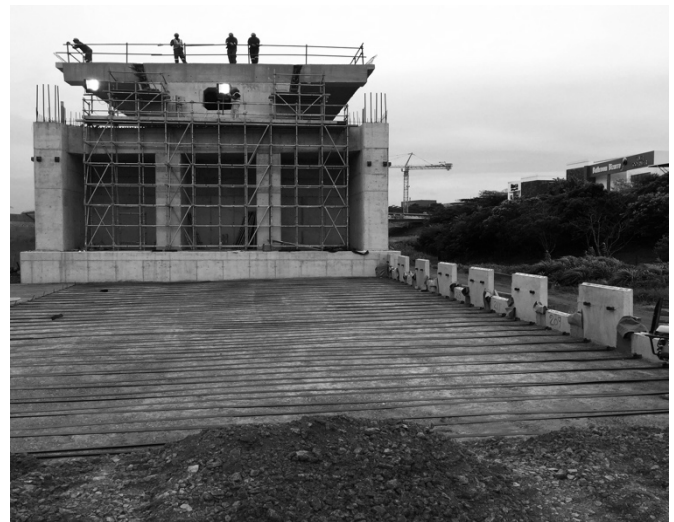
Figure 3. Back-to-back MSEW at one of the Viaduct Abutments
