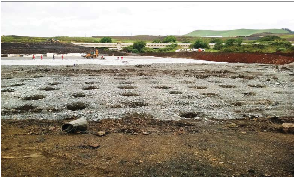
Ground improvement comprising dynamic replacement craters
