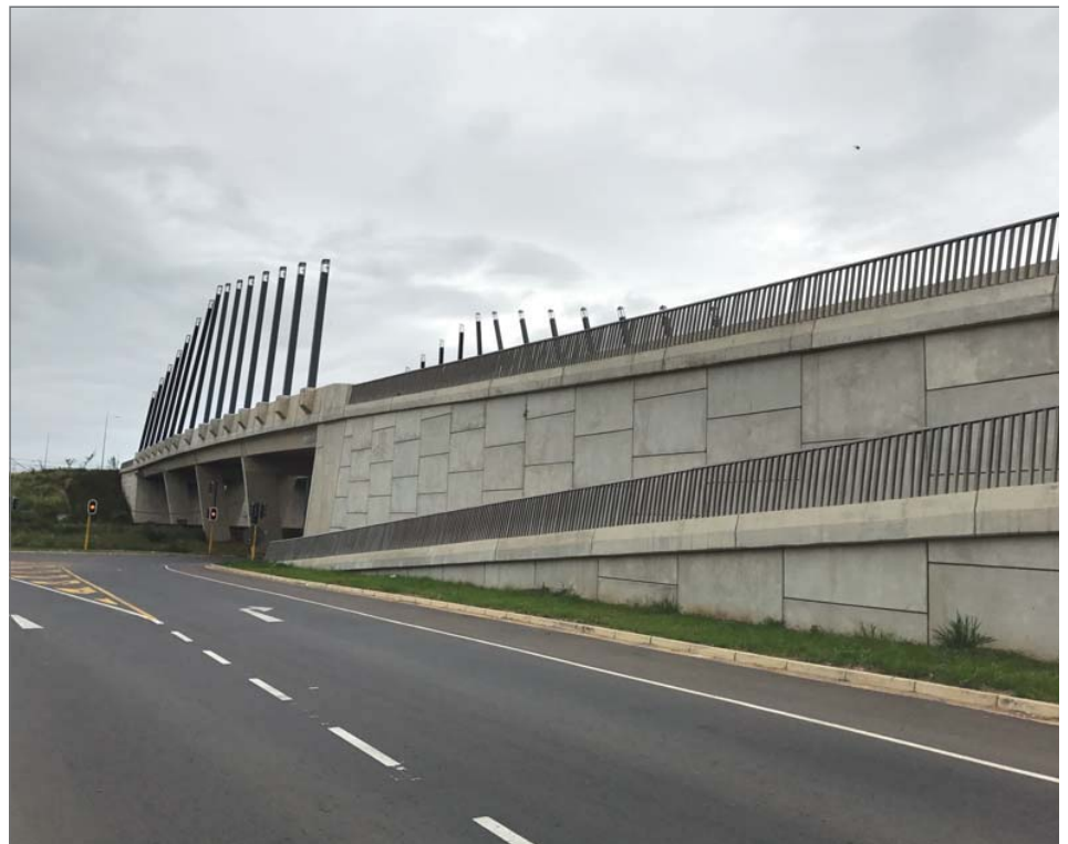
Completed Cornubia Bridge and MSE walls – MSEWs are the ultimate geotechnical structures, as they have an incontrovertible link with the soils within, around and below
